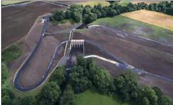
The scheme opened in August 2015, at a cost of £26m. It includes one of the largest flood storage reservoirs the Environment Agency has ever built and reduces the risk of flooding to 1000 homes and businesses in the area. The upstream dam and storage area work by storing up to 1.4 million cubic metres of water when river levels are high. There is now a 0.7% chance of river flooding in Morpeth each year. The scheme created 17 hectares of new habitat for local wildlife.
